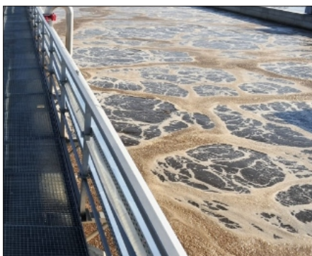
Wastewater Treatment Power Generation
